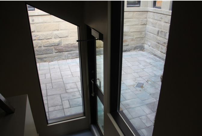
The new courtyard, with improved drainage and the staircase leading to the Library's basement storage.
