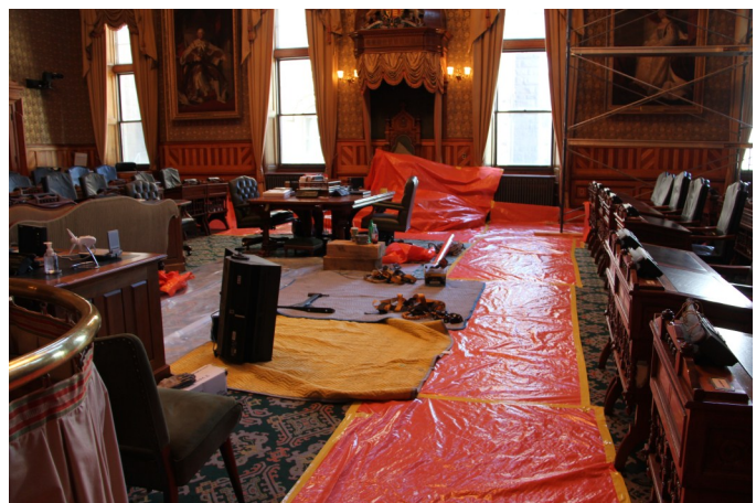
In September 2011, contractors proceeded with the removal of eight large fluorescent lights in the Legislative Chamber.
