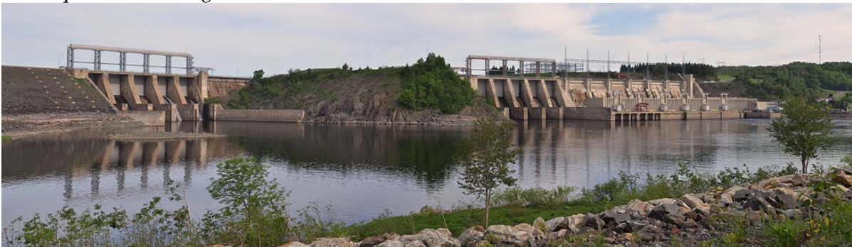
Mactaquac Generating Station
