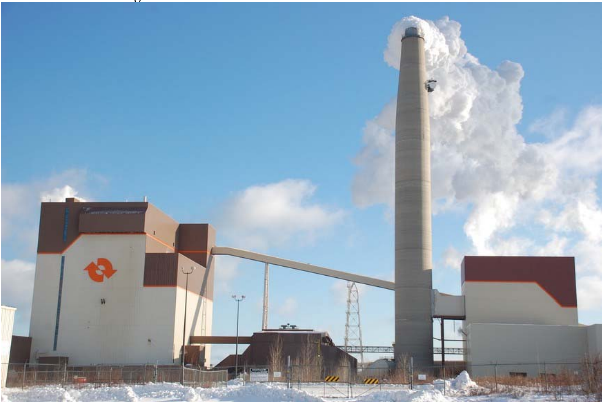
Belledune Generating Station
