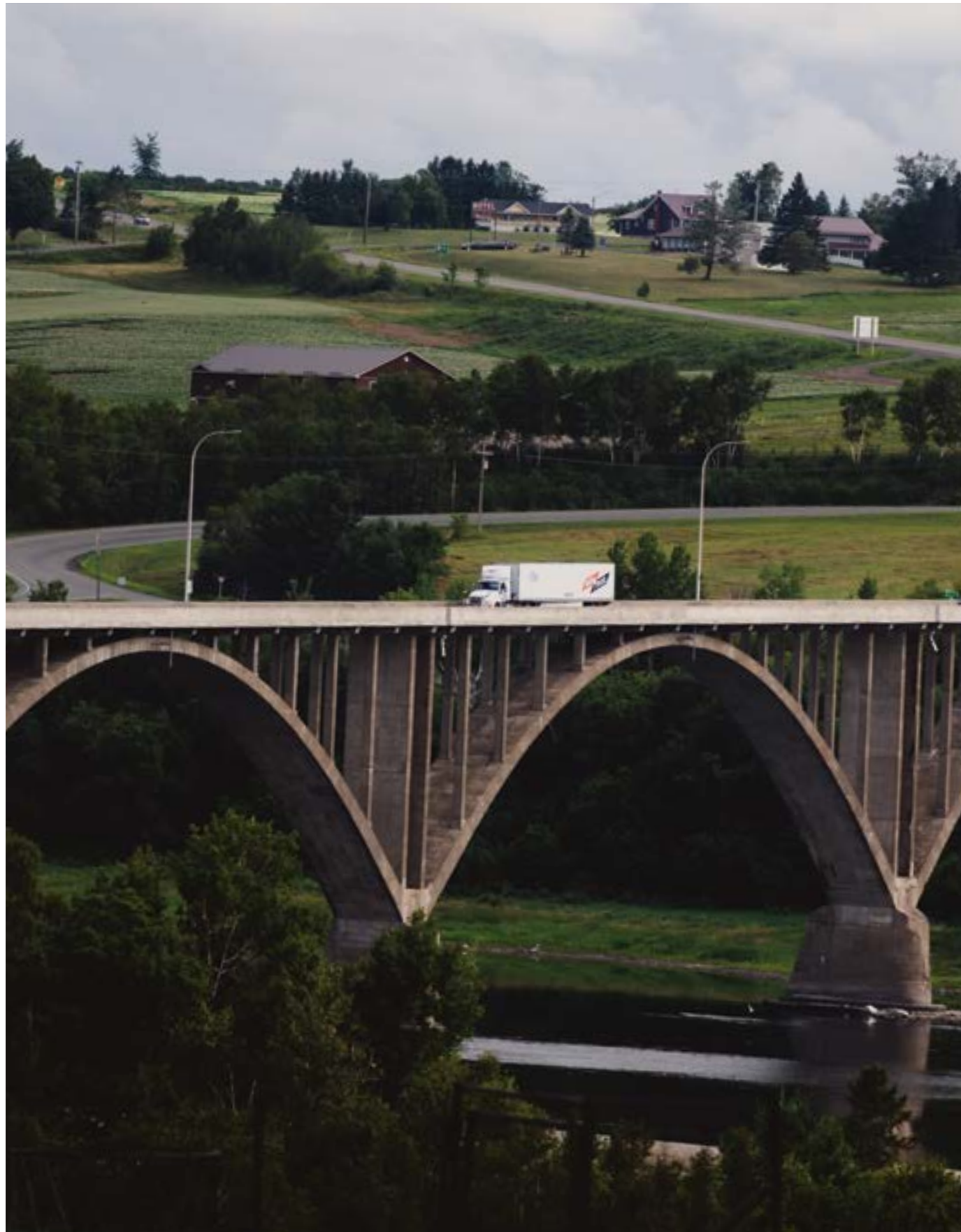
Hugh John Flemming Bridge, Hartland, New Brunswick
